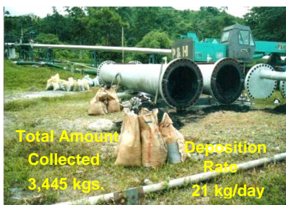
Figure 12: Modified Solid Trap installed at W1R8D
