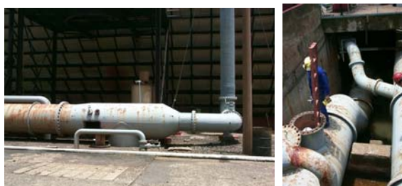
Figure 3: Locations for access to Hot-Side CW pipelines, at vertical T (at left photo), manhole to subsurface straight pipe section (at right photo). Cold-Side CW pipeline is seen at right of right photo.
