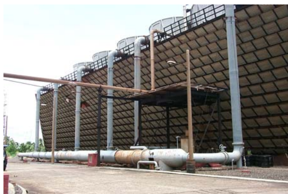
Figure 2: MakBan Plant C Unit 6 cooling tower and Hot Side CW distribution and riser pipelines.
