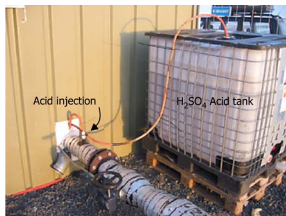
Figure 13: Acid tank and acid injection at well ÓS-1.
