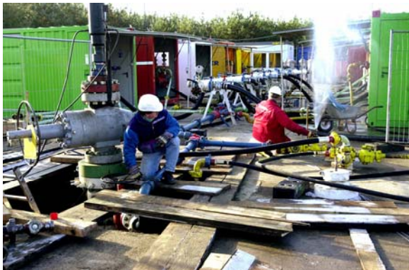
Figure 3: Impression from the stimulation experiments: wellhead with riser in front, ten high pressure pumps (HT400) with low and high pressure manifold in the back (photo by A. Weitze).
