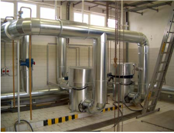
Figure 11: Coarse filtration of the thermal water at the “cold” well
