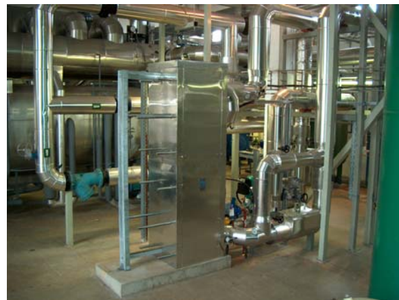
Figure 10: Heat exchanger between district heat supply network and intermediate loop
