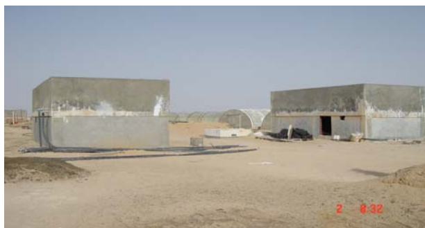
Figure 8: Concrete Ponds for Irrigation
