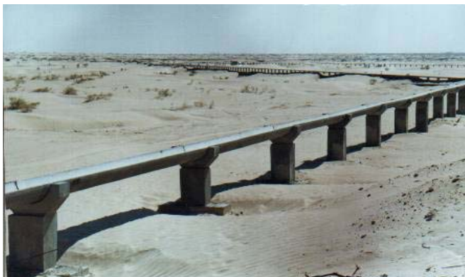
Figure 4: The concrete canalization for oasis irrigation (Douz project)
