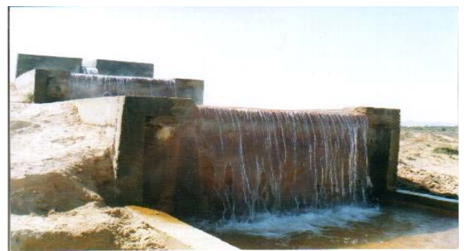
Figure 3: The Water Cooling System (Cascade of Oum Elfareth)
