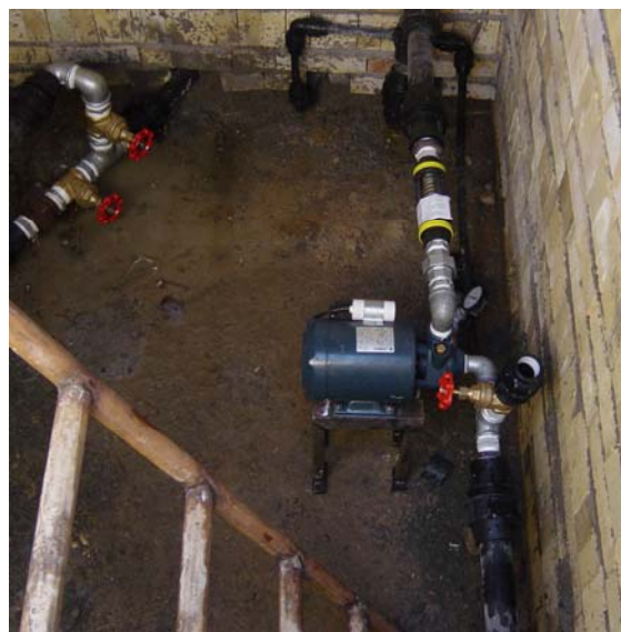
Figure 3: Installed circulator pump.
