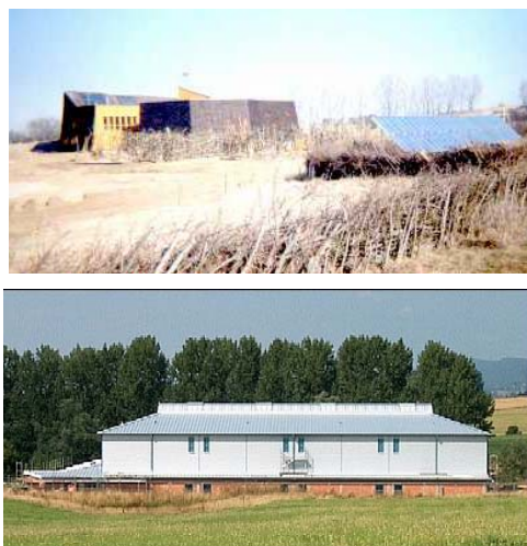
Figure 23: GSHP-plants with solar recharge; natural park information centre “Blumberger Mühle”, with solar panels in the right foreground (above, photo GTN) and gym in Hessisch-Oldendorf, with solar collectors (below, photo EWS)
