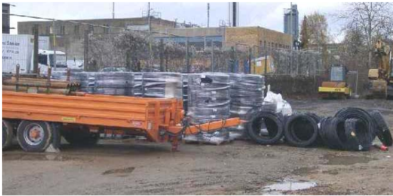
Figure 6: Factory-made BHE in coils at the site in Wetzlar-Spilburg (photo UBeG, Nov. 2004)
