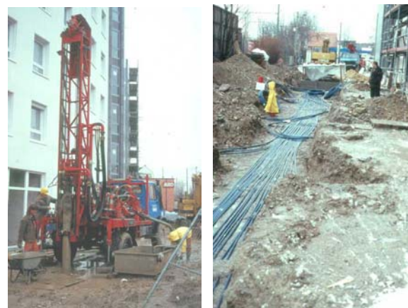
Figure 29: Drilling for shallower BHE in Frankfurt-Hoechst, and connecting pipes (photos Sanner)
