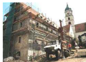
Figure 24: Drilling for BHE at the town hall in the historic centre of Unlingen (photo Systherma)
