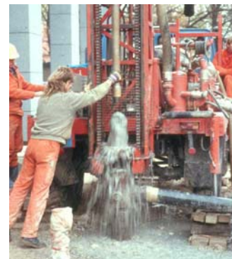
Figure 28: Artesian water flow from drilling in Frankfurt-Hoechst, 1993 (photo Sanner)
