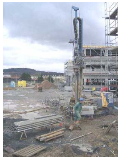
Figure 5: Drilling of the 4 th borehole for the plant in Wetzlar-Spilburg; an already installed and grouted BHE can be seen in the right foreground, the borehole field will extend towards the earth mound in the background (photo UBeG, Nov. 2004)
