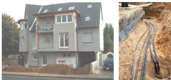
Figure 18: Apartment house in Frechen and head of a BHE with connecting pipes (photos EWS)
