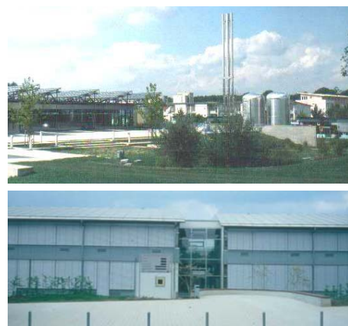
Figure 39: System concept of Neckarsulm BTES (graph after ITW); below view to the gym with solar collector on the roof and accumulator tanks right, and school with roof-integrated solar collectors (photos Sanner)
