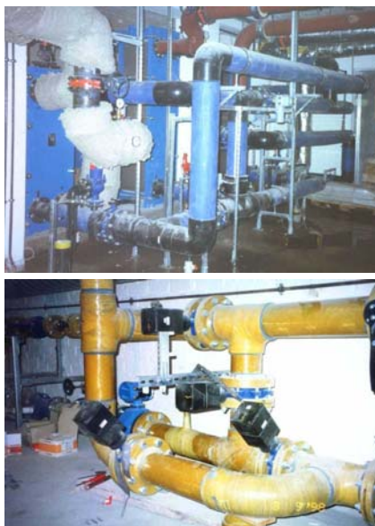
Figure 6: Groundwater-bearing pipe connections at the entrance into the Reichstag building, cold storage system (above) with heat exchangers to the left, and heat storage system (below) (photos: GTN)
