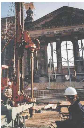
Figure 3: Drilling of the first deep well in front of the main entrance in 1996, while the complete interior of the building has been removed before rebuilding (photo: GTN)
