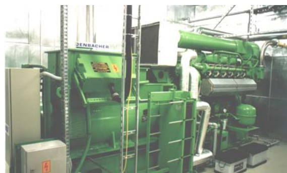
Figure 6: Co-generator unit (Jenbacher, 0.54 MW e + 0.7 MW t ) in the Podhale geothermal plant.
