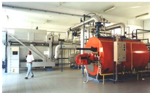
Figure 5: Absorption heat pump (Sanyo, 2.7 MW) co-operating with high-temperature boiler (Viessman, 1.9 MW) in Mszczonów geothermal plant.
