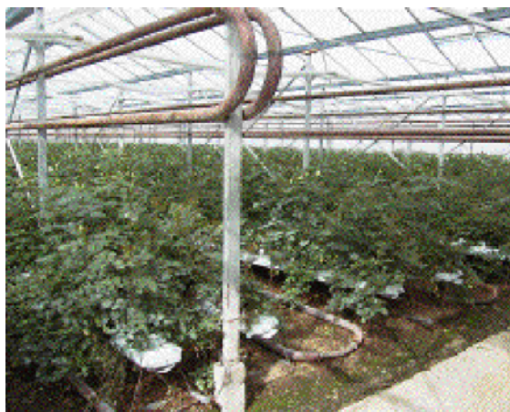
Fig. 10. Location of heating pipes in greenhouses (high and low temperature system)
