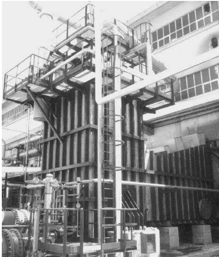
Figure 5: Direct Contact Condenser During Installation
