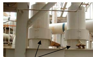
Figure 7: General view of the mesh demister
