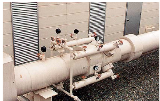
Figure 11: General view of the venturi tube
