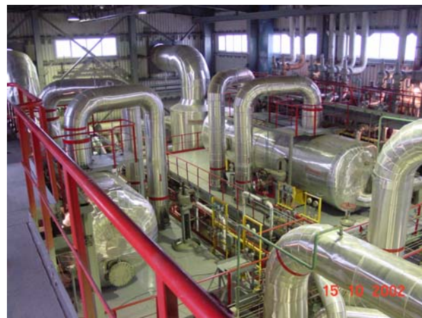
Fig. 6 I stage separators of Mutnovsky GeoPP in separator building.
