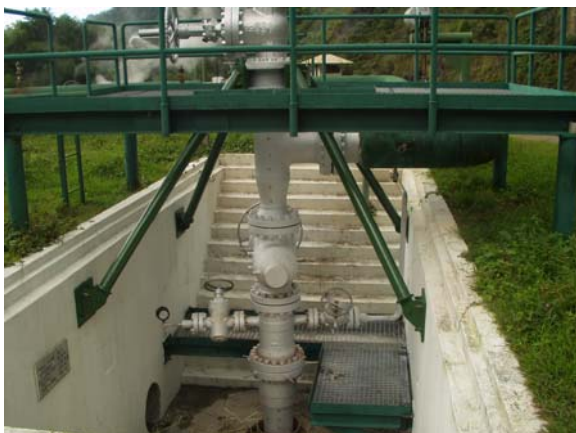
Figure 5: The Rehabilitated Well OK5
