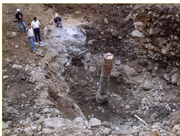
Figure 9: The topmost cut-off casing of Well 5R-12D
