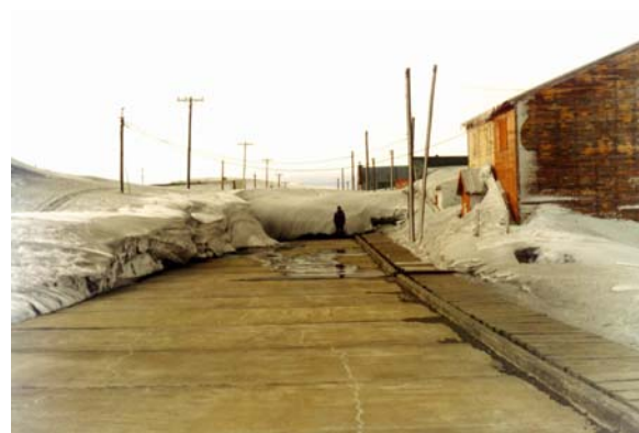
Figure 4: A street in Copahue village showing the geothermal heating system.
