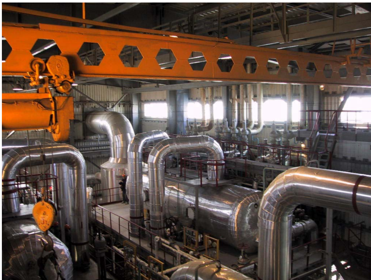
Figure 7,b. Mutnovsky GeoPP. Primary separators provide MGeoPP with the high-quality steam. Photo of Svalova V.B.
