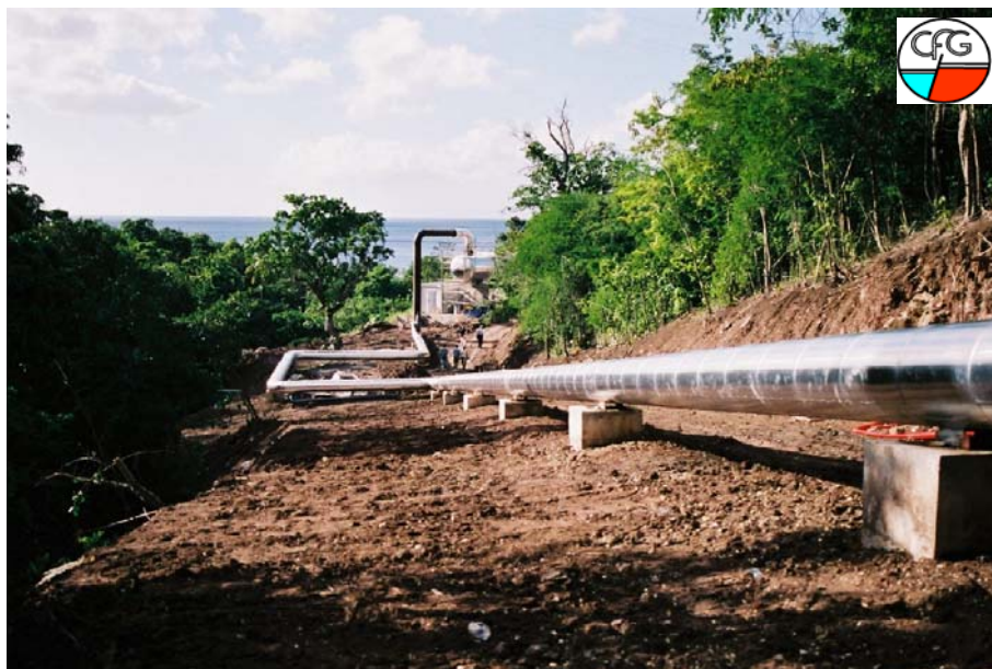
Figure 6: Steam supply lines at Bouillante 2
