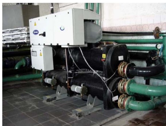
Figure 6: Heat pump installation in a water-supply station near Minsk, Zhidovich and Belvi (2003).
