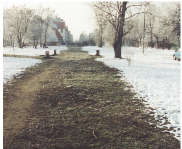
Fig. 5. Heat escaping from insufficiently insulated, district heating, delivering pipes could be easily utilized in direct-use snowmelt systems, without additional producer cost. A heating-pipe course in Warszawa, Poland, after the night snowfall. Winter, 1998/99; outside temperature -12^{\circ}\text{C} ( 12^{\circ}\text{C} below freezing point).
