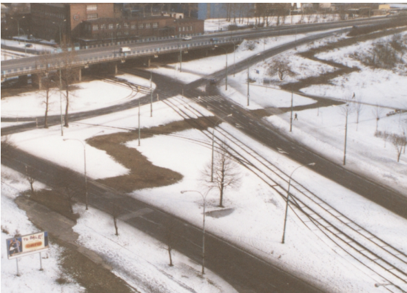
Fig. 8. Zigzagging path of a district heating power-line, and salted asphalt roads look very alike except that asphalt is wet with highly corrosive brine. Sosnowiec, Poland; -8^{\circ}\text{C} ( 8^{\circ}\text{C} below freezing point).
