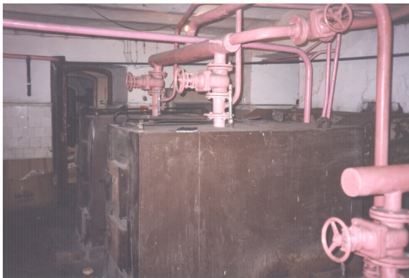
Fig. 3. Old-fashion, low efficiency central heating boiler; one of many open furnace, coal powered pollutant.
