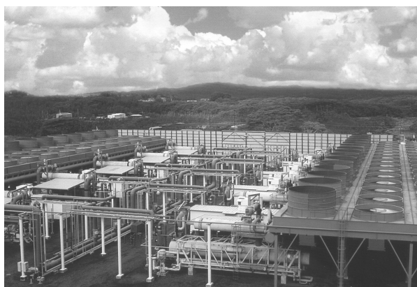
Figure 4. Puna Geothermal 30 MW Air Cooled, Combined Cycle Power Plant
