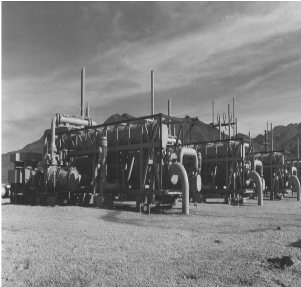
Figure 6. Empire Geothermal 4.8 MW Water Cooled Binary Power Plant
