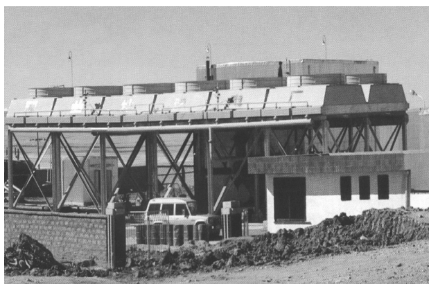
Figure 8. Nagqu 1.3 MW Air Cooled Binary Power Plant
