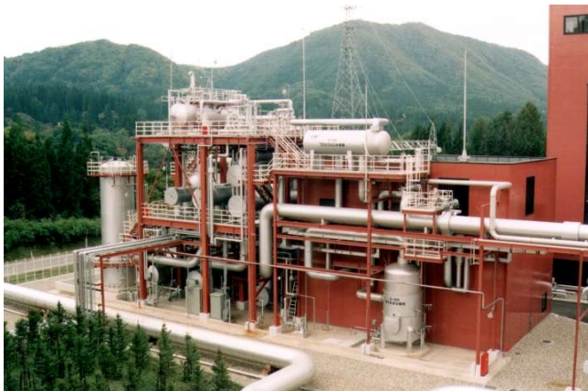
Photo 3 Dry-type hydrogen sulfide abatement system
