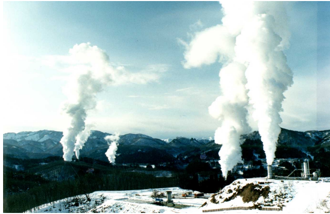
Photo 1 Well flow test at Yanaizu-Nishiyama Geothermal Power Station. Well flow steam normally diffuses upward.
