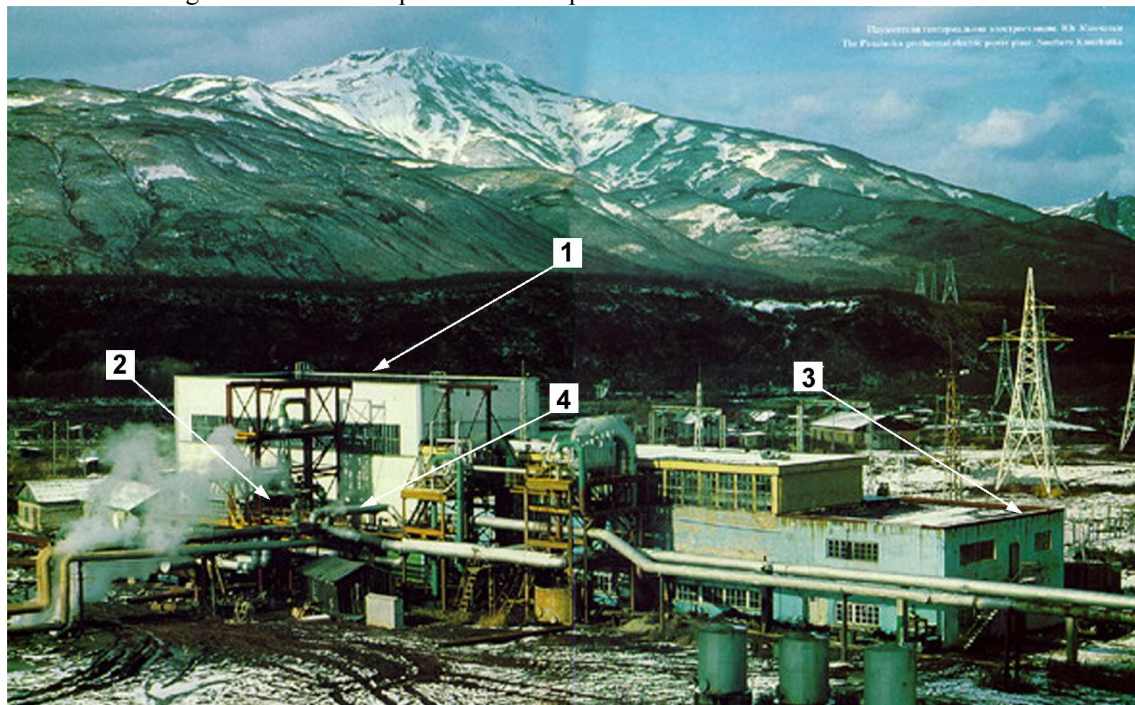
Figure 3. Pauzhetskaya GeoPP (1965) 1—power unit; 2— wet steam supply ( p_0 \approx 4 bar); 3— administrative building and laboratory; 4— geothermal heat input.
