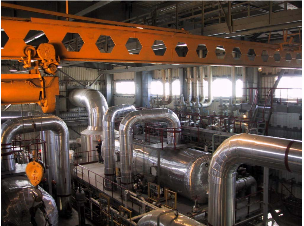
Figure 4,b. Mutnovsky geothermal power plant (MGeoPP). Primary separators provide MGeoPP with the high-quality steam. Photo of Svalova V.B.
