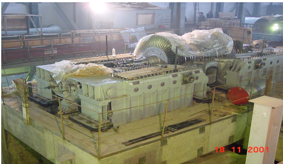
Figure 1. Erection of type K 25-0.6 Geo Turbine at the Mutnovsky GeoPP.
