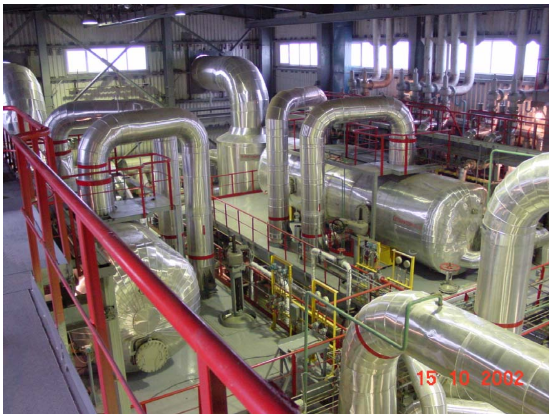
Fig. 4 I stage separators of Mutnovsky GeoPP in separator building
