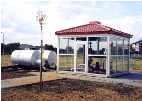
Figure 16. Geothermal intake (extraction well) in geothermal plant in Uniejow
