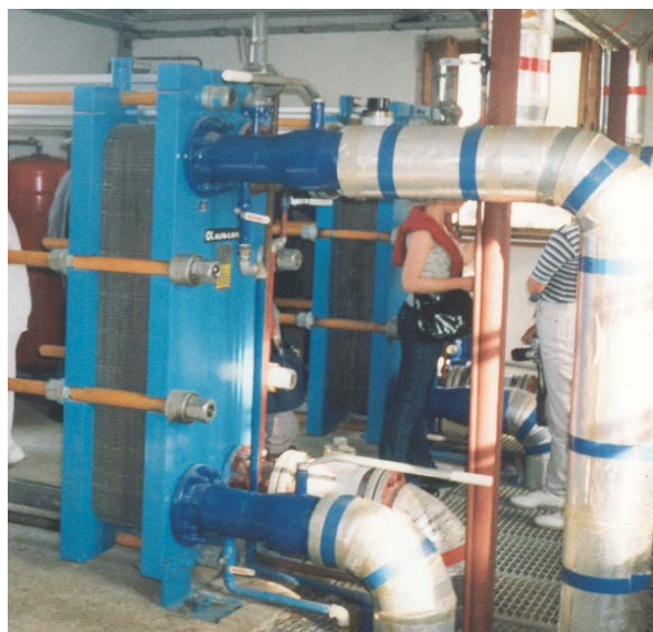
Figure 4. Geothermal heat exchanger in geothermal plant in Banska
