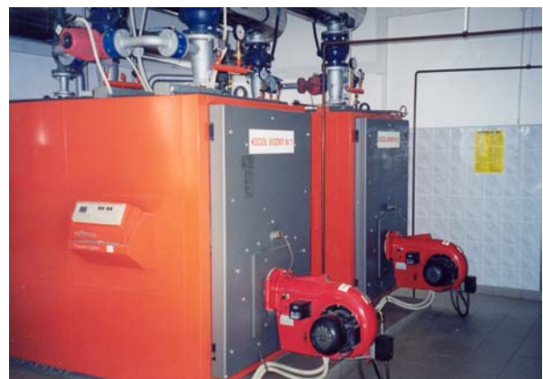
Figure 19. Gas peak boilers in geothermal plant in Uniejow
