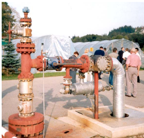
Figure 3. Geothermal intake (extraction well) in geothermal plant in Banska
