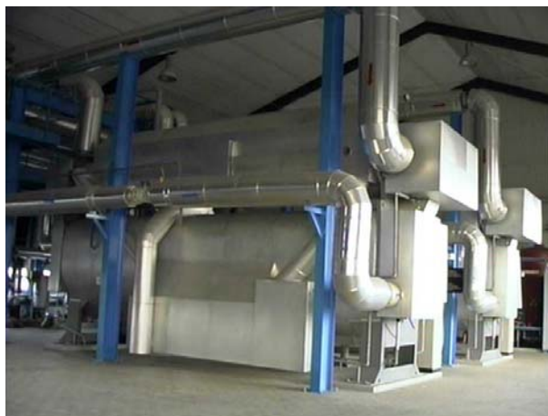
Fig. 11. Absorption heat pumps in geothermal heat plant in Pyrzyce
