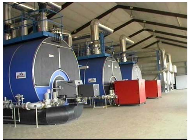
Fig. 12. High and low-temperature gas boilers in geothermal heat plant in Pyrzyce
