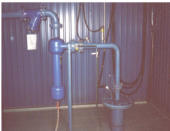
Figure 14. Geothermal intake (extraction well) in geothermal plant in Mszczonow
