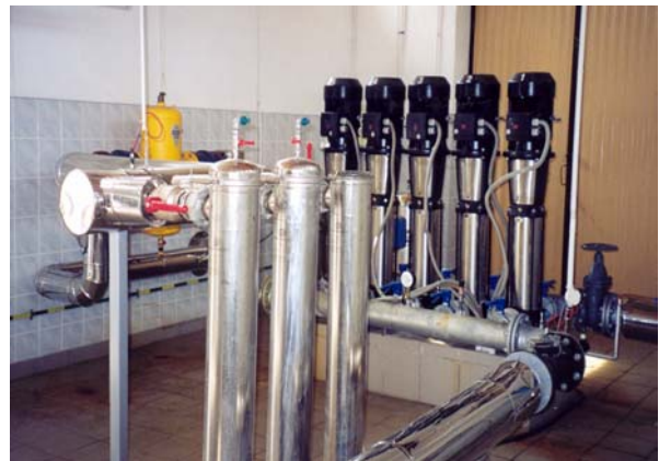
Figure 17. Pipeline with geothermal water, filters and injection pumps
