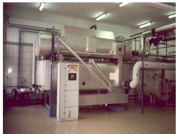
Figure 15. Absorption heat pump in geothermal plant in Mszczonow
