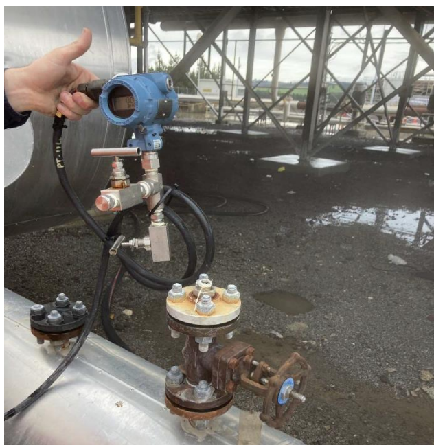
Figure 12: Loose pressure instrument tubing connection
