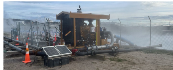
Figure 16: Pumping hot brine with a large centrifugal pump.
