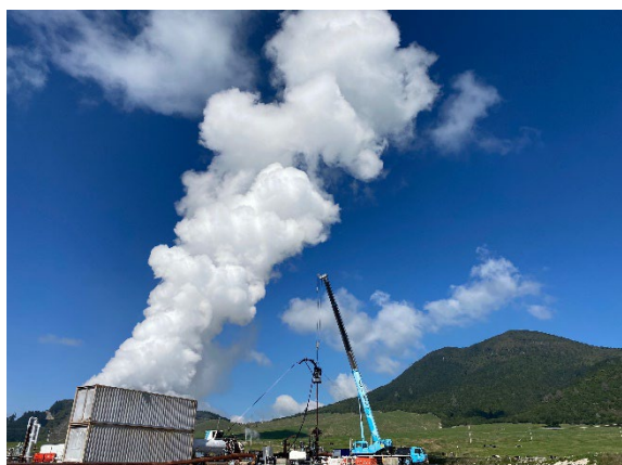
Figure 1: Well test initiated by coil tubing air lift on Tauhara Steamfield, Taupo, New Zealand.
