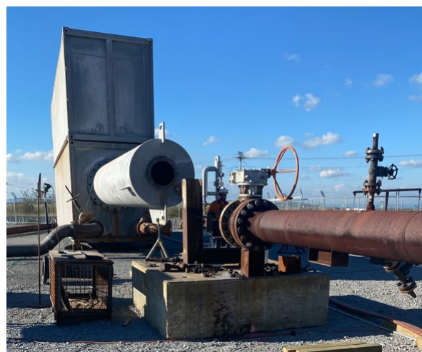
Figure 4: LECM with S-Bend removed post pinhole failure.
