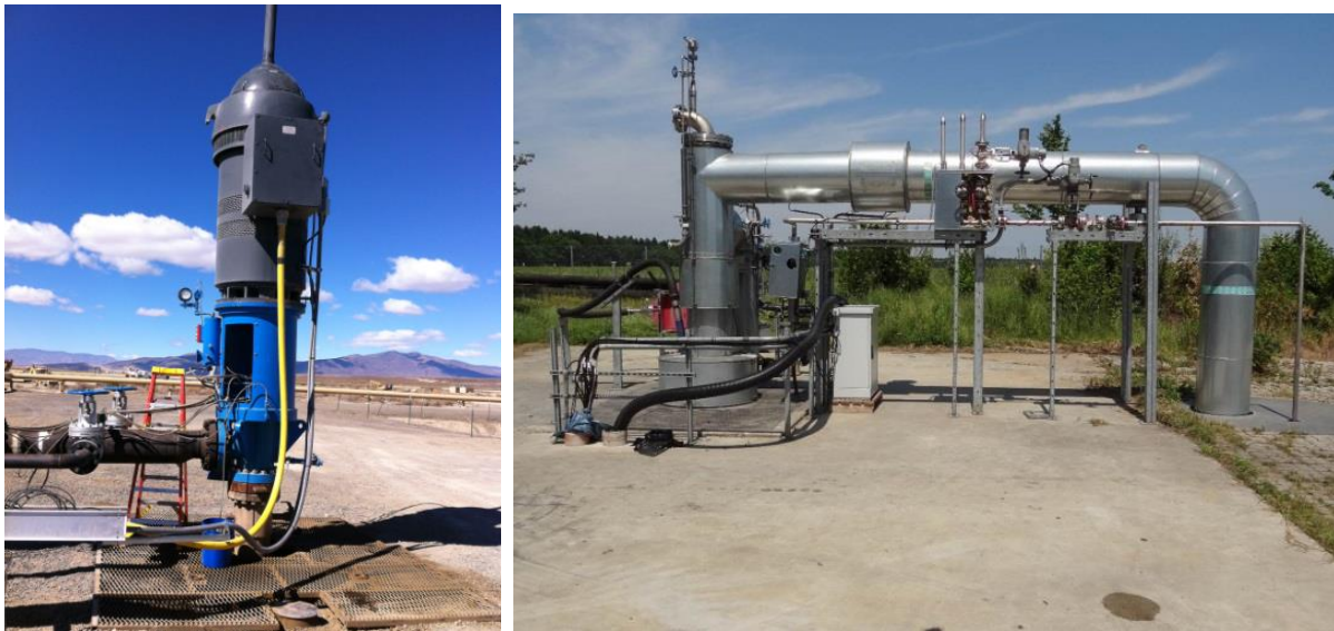
Figure 3 Lineshaft pump installed at a well in USA (Left, the motor is visible, but the pump is down the well). ESP installation in Germany (Right, wellhead arrangement shown – ESP itself not visible as it is installed in the well)
