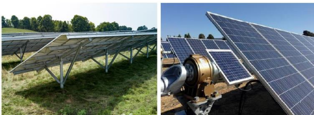
Figure 2: Fixed tilt (left) and single-axis tracker (right) systems used in ground-mounted solar PV systems
