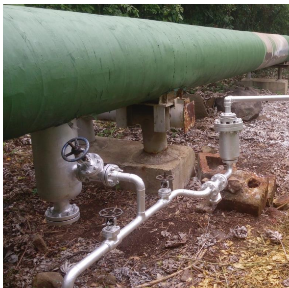
Figure 3: Typical Condensate Drain Pot with Inverted Bucket Steam Trap Arrangement.
