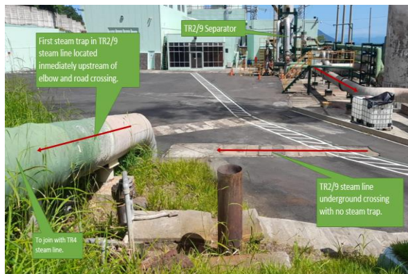
Figure 15 - TR-2/9 Steam Line and Road Crossing
