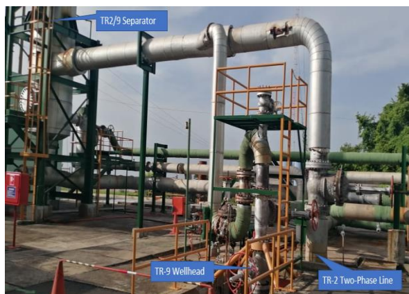
Figure 16 - Two-Phase Inlet at TR-2/9 Separator
