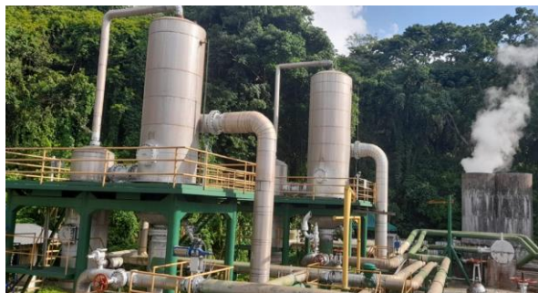
Figure 2: Separation Station at TR-4 Production well pad (see Figure 1)
