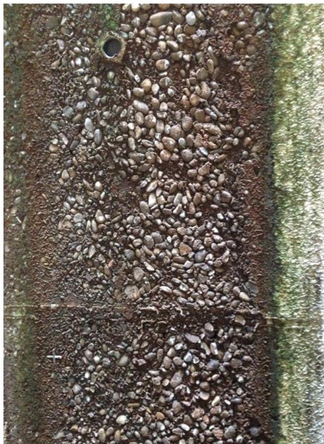
Figure 9: Example of more severely attacked vertical area of tower shell, approximately 300 mm wide (2018 outage inspection)
