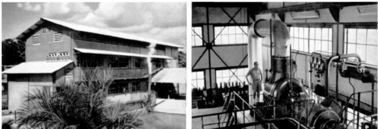
Figure 5: Kiabukwa power plant showing the powerhouse (left) and power island (right) [Source: DiPippo 2015 taken from Rollet 1957]
