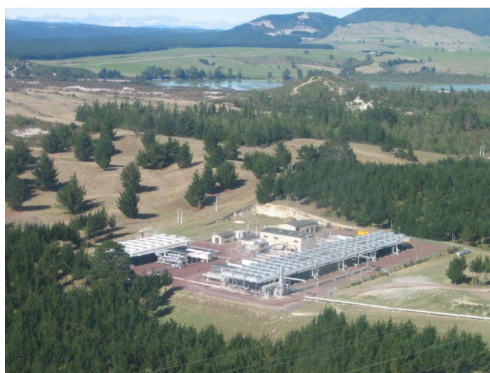
Figure 1. An early photo of the Rotokawa Power Station, with Lake Rotokawa and Mount Tauhara in the background. OEC21 is located to the left of the plant site. The Production line running to the original vertical separator is from the right.
