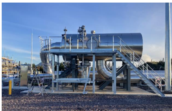
Figure 6. Photo of the newly completed H-Line Separator (two-phase inlet from right)
