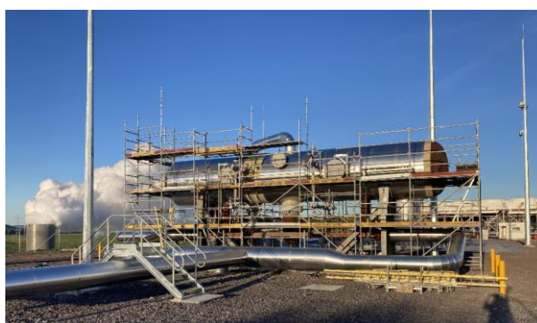
Figure 8. Photo of the near-complete Rotokawa Separator (insulation is partly complete), Two-phase inlet from the left
