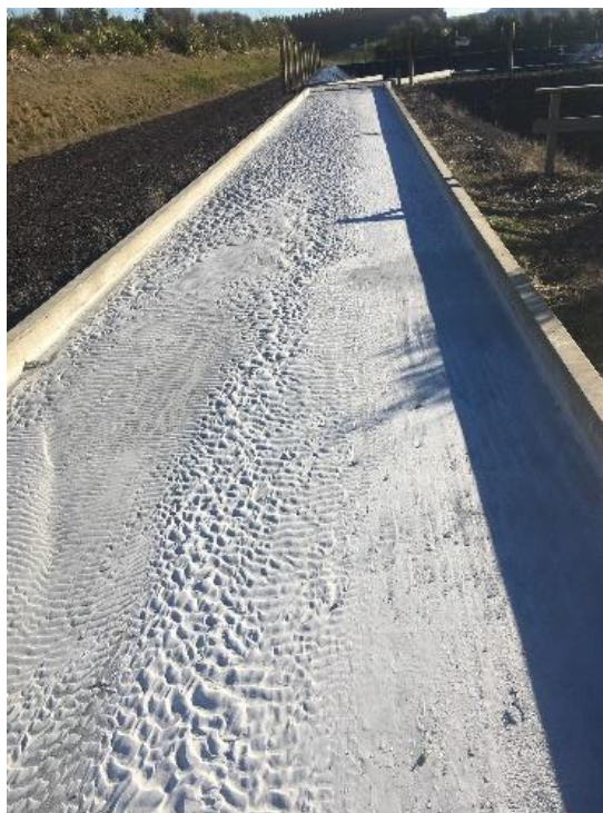
Figure 1: Cooling channel lined with fragments of calcite scale removed from a production well with live well cleanout technology.
