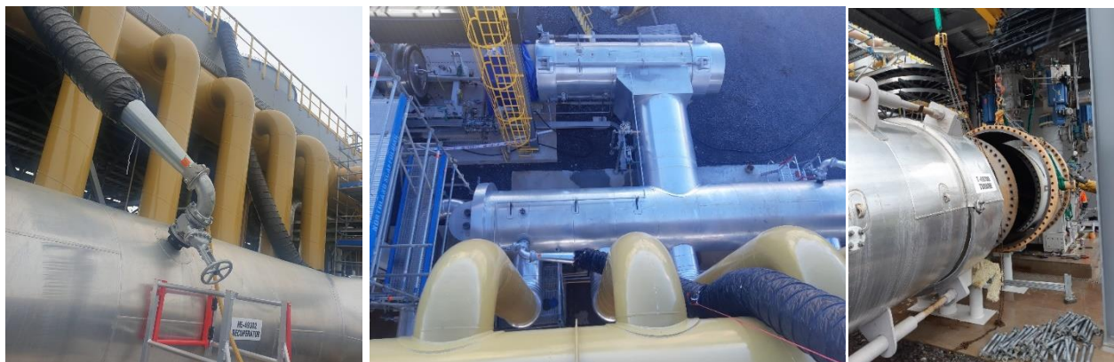
Figure 7: Left- Venturi, ducting and isolation valve installed on inspection hatch. Middle- Turbine halfway through repairs, with two Venturi eductors and ducting still in place. Right - Spool piece being removed ready for blank flange install.
