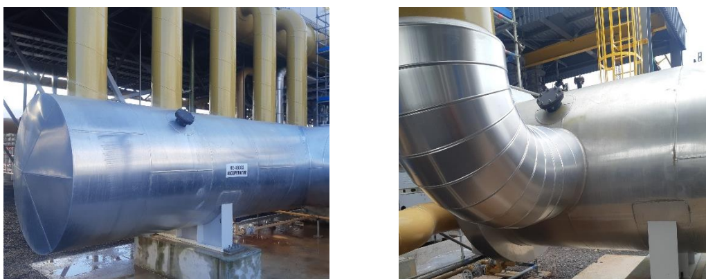
Figure 5: Location of 6" CL150 Inspection hatches on recuperator
