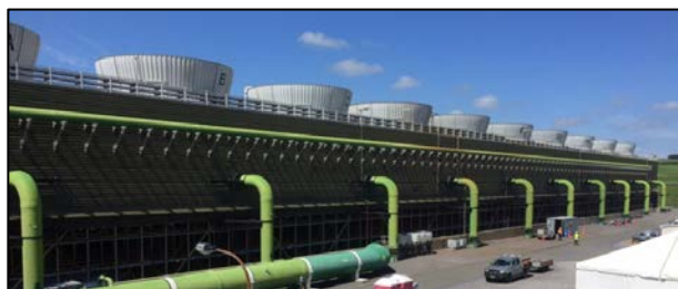
Figure 2: Cooling Tower at Nga Awa Purua Power Station (cells A to F run from left to right in photo)
