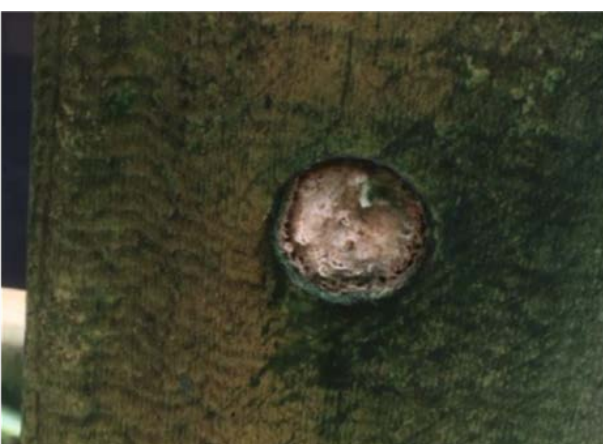
Figure 4: Examples of FRP degradation in the tower zone above the Drift Eliminator layer
