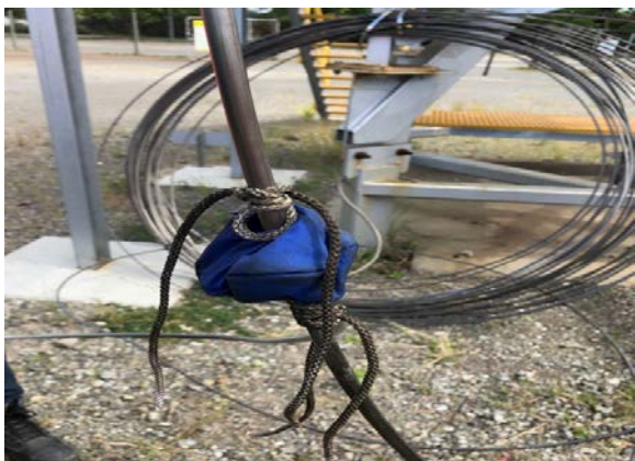
Figure 4: Ice bag on the anti-scalant tubing
