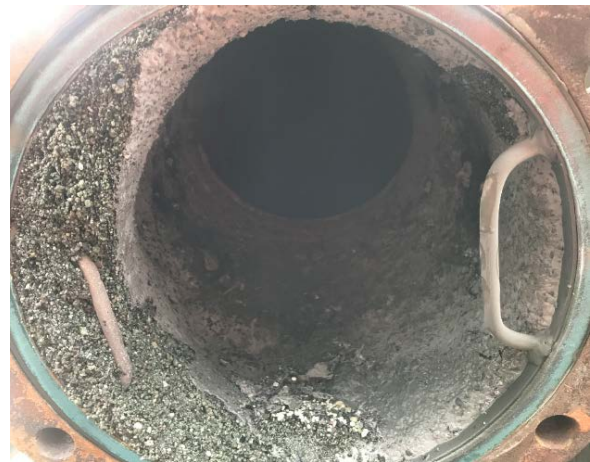
Figure 1. Debris from geothermal well in a blocked strainer.
