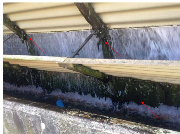
Figure 4: Algae growth on side of cooling tower.
