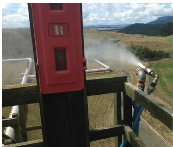
Figure 5: Aerosol emitted during algae removal.
