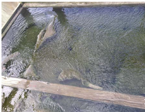
Figure 3: Algae growth on open top deck water distribution boxes of cooling tower just prior to cleaning.
