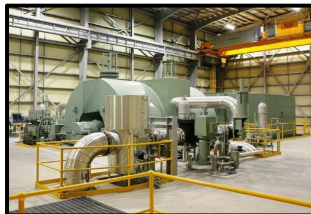
Figure 4: Geothermal Direct Contact Steam Turbine
