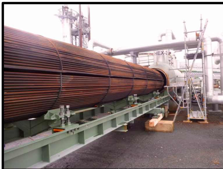
Figure 4: HEX 2 Tube Bundle Inspection – Late 2018 – Obvious Surface Corrosion Evident
