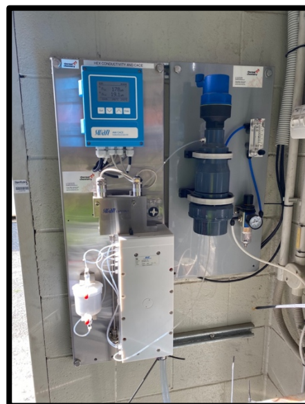
Figure 10: SWAN AMI CACE Analyser (right) with Geothermal Specific Modifications (left)
