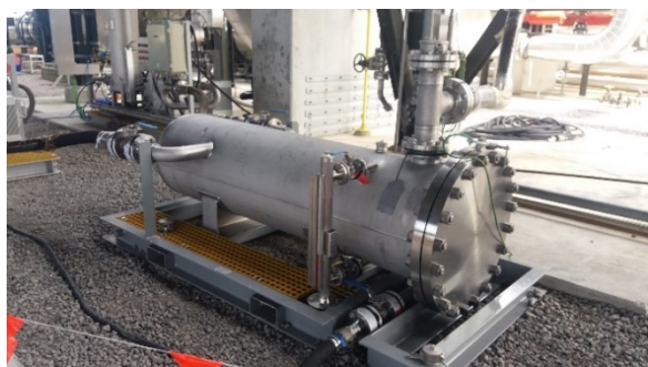
Figure 11: Vacuum pump exhaust collection vessel allows condensed pentane in the vacuum pump exhaust line to be safely recovered.
