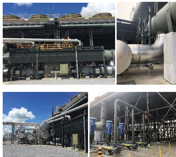
Figure 3: Photos of an OEC at the Ngatamariki Power Plant from top left: Turbines, Turbine Exhaust Piping, Feed Pumps; and Heat Exchangers
