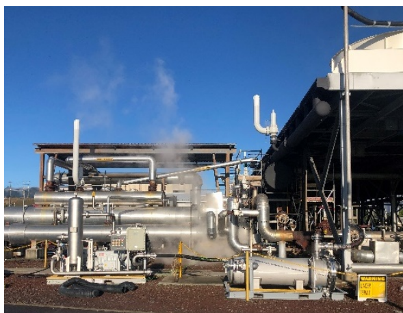
Figure 12: Pentane Evacuation Skid and Exhaust collection vessel installed at Rotokawa Power Plant OEC01 unit.
