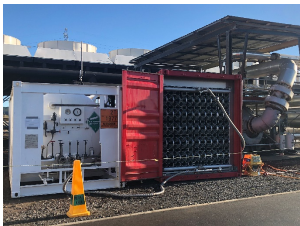
Figure 4: Liquid nitrogen supply and vaporiser in use at Rotokawa Power Station
