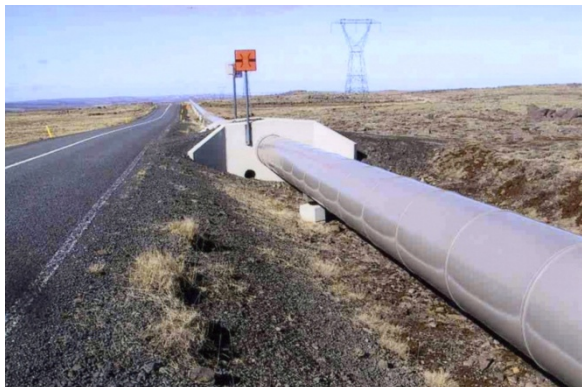
Fig. 1: Hot water pipeline (transport system) seen from the ground surface. Note the size of the pipe, the roadside ditch the pipe is housed in and a small bridge for snowmobiles (beige, by the sign). The whole area is snow-clad for most of the year (©Katherine Luketina).
