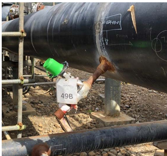
Figure 5: Brine sampling point, a cooling coil was connected to the point for brine sampling.
