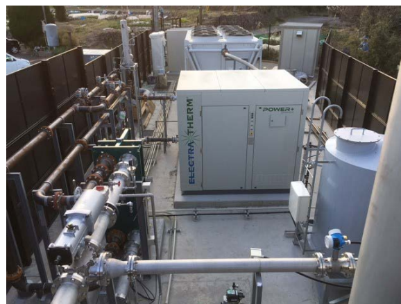
Figure 6: ORC Installation at Beppu Japan
