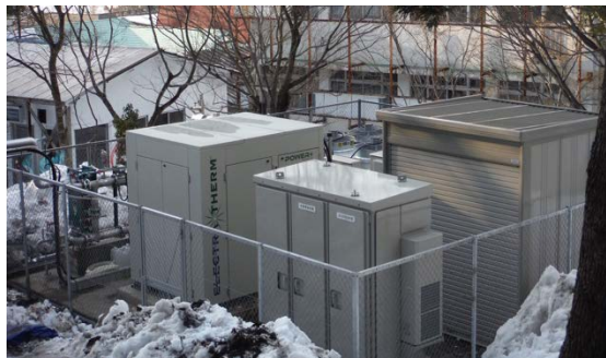
Figure 7: ORC Installation Central Japan
