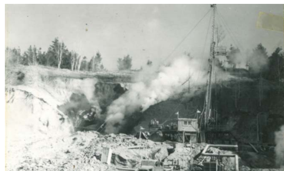
Figure 1: Rig sitting over WK26 with a blowout crater in the background that was the result of an untreated casing breach
