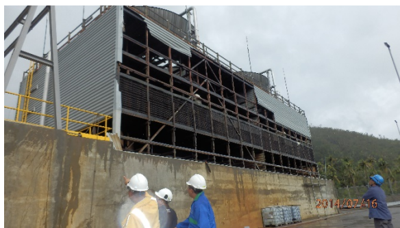
Figure 3. Cooling tower sidings of 20MW Maibarara-1 plant blown away during Typhoon Glenda in July 2014.
