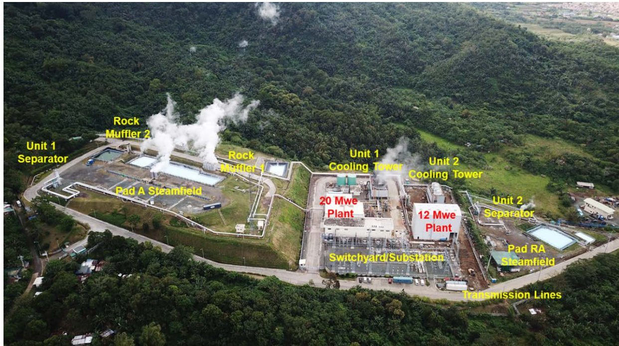
Figure 1. Overview of the 32 MW Maibarara geothermal facility, looking southwest. Extent of development is 613 m long (from left to just outside the right edge of photo) to 150 m wide (at center of photo). Note heavy tropical forest vegetation enclosing much of the facility which has an areal footprint of 9 hectares.
